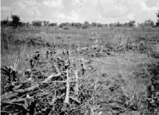
A- These pictures show a close up of the brushwood gabion. To the right of the gabion the silt has been trapped, and prevented from entering the spring -- which is to the left of the picture.
